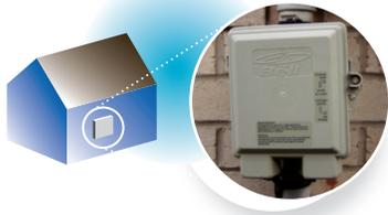
Locate your telephone Network Interface Device (NID). This is usually a grey plastic box on the outside of your home where telephone service enters. It may also be in your basement or garage. This box is a demarcation point between the phone network, owned by the local phone company, and your home wiring, owned by you.
