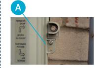
Open the "customer"side of your NID (A). You should see one or more phone lines plugged into phone jacks (B) or one or more sets of wires connected to terminals (C); these are the phone lines coming into your home. If you have one phone line there will be likely be only one connection.
